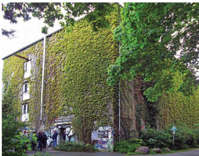
The daunting facade of the Eidelstedter Weg bunker, softened with Virginia Creeper which is reminiscent of Brislington bunker near Bristol. The gantry and loading doors were added postwar when the structure was used as a warehouse. Photo Adrian Armishaw
